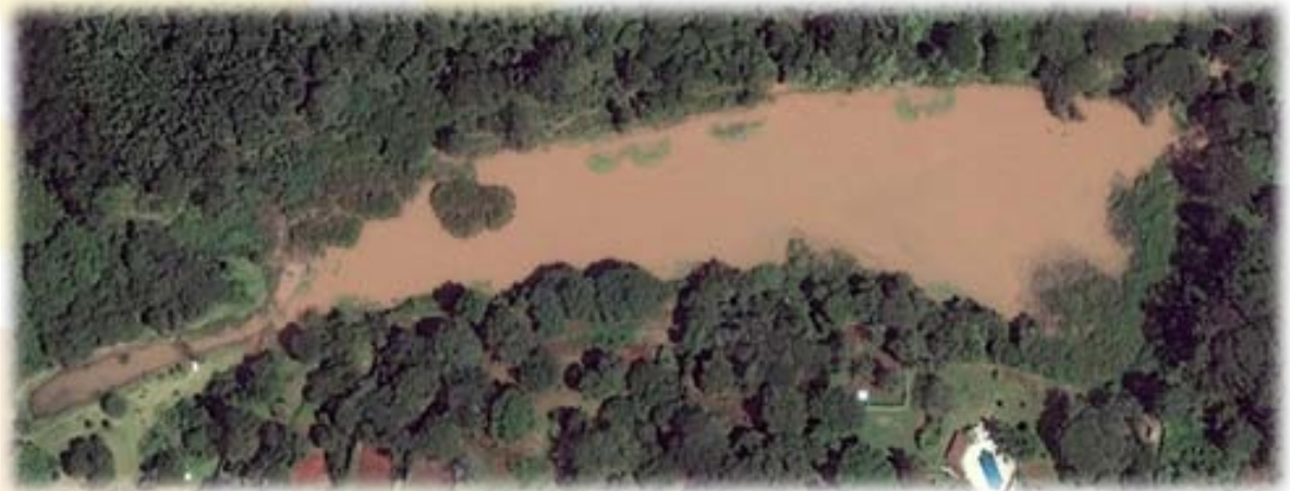
Aerial view of the Lower dam in Section 1 of the Ngong Road Forest
