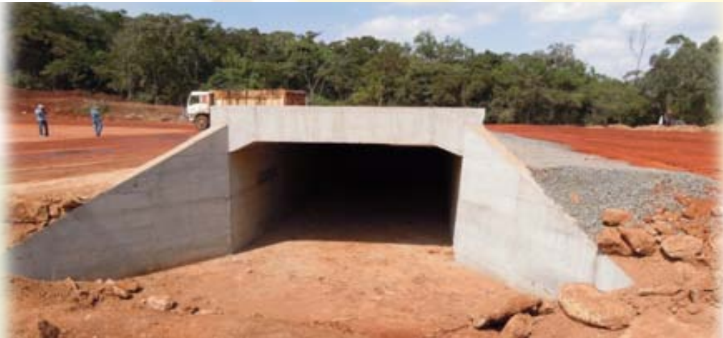
Construction of the Underpasses along the Southern Bypass
