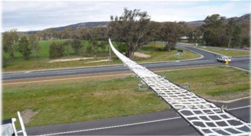
Illustration showing a Proposed Rope Bridge along the Southern Bypass
